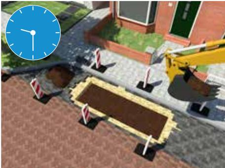
Placing (15 cm) of water-permeable granulate/soil.
