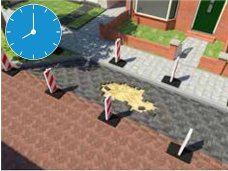
Removing the paving in the parking spaces.
